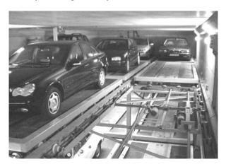
A vertical transport system moves the pallets to the various parking layers and/or to and from the admission room facing the right direction for leaving the room.
