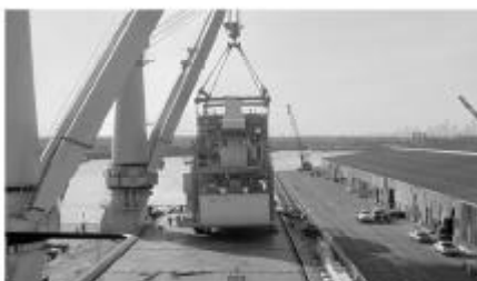
Vessel crane loading compressor module in a single lift on board
