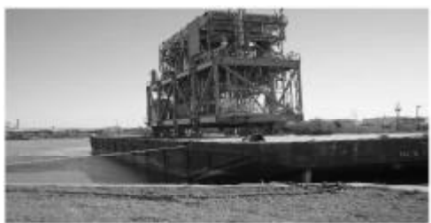
Loading of compressor module on barge
