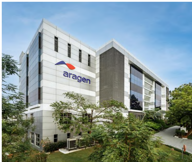
Our facility at Nacharam, Hyderabad
