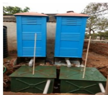
FRP Toilet With Bio-Digester Tank
